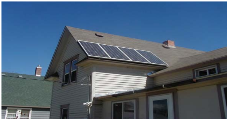
Solar Panels on Powder River Main Office
