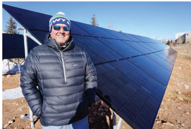
ARE member and Technical Solar Salesman Leo Pueblitz stands next to a new array that serves power to the Laramie Community Recreation Center and the Ice & Event Center. Photo credit: Creative Energies.
